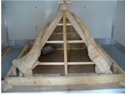
Fig. 2 Glasswool applied between rafters
