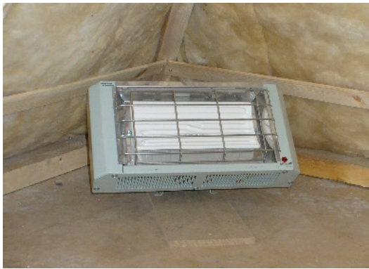
Fig. 8 Ceramic heater in position
