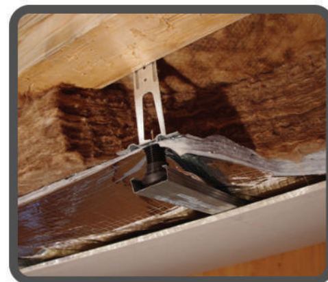
SIXBOX hangers to ensure seal
